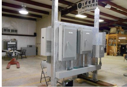
PLC PANEL ON SWITCH RACK – PIPELINE LOCATION
